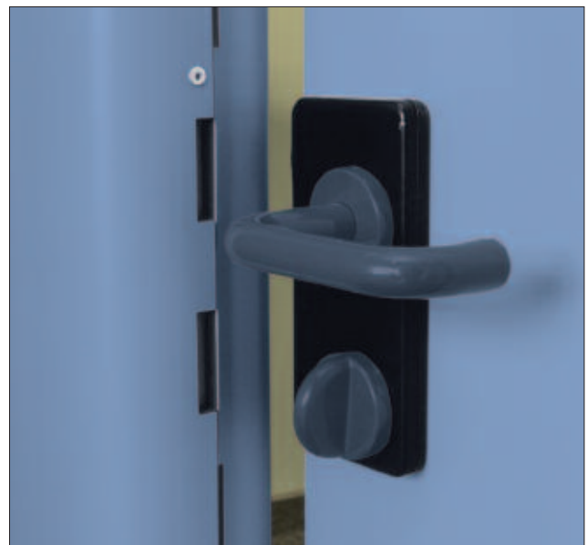
Lock socket with striking plate
